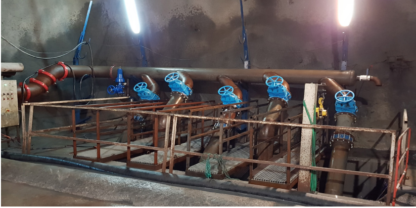
Tunnel EURALPIN - FRANCE
