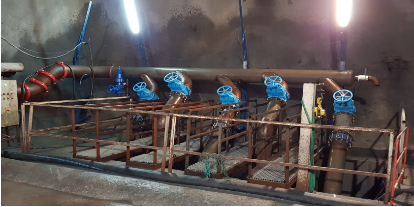
Tunnel EURALPIN - FRANCE
