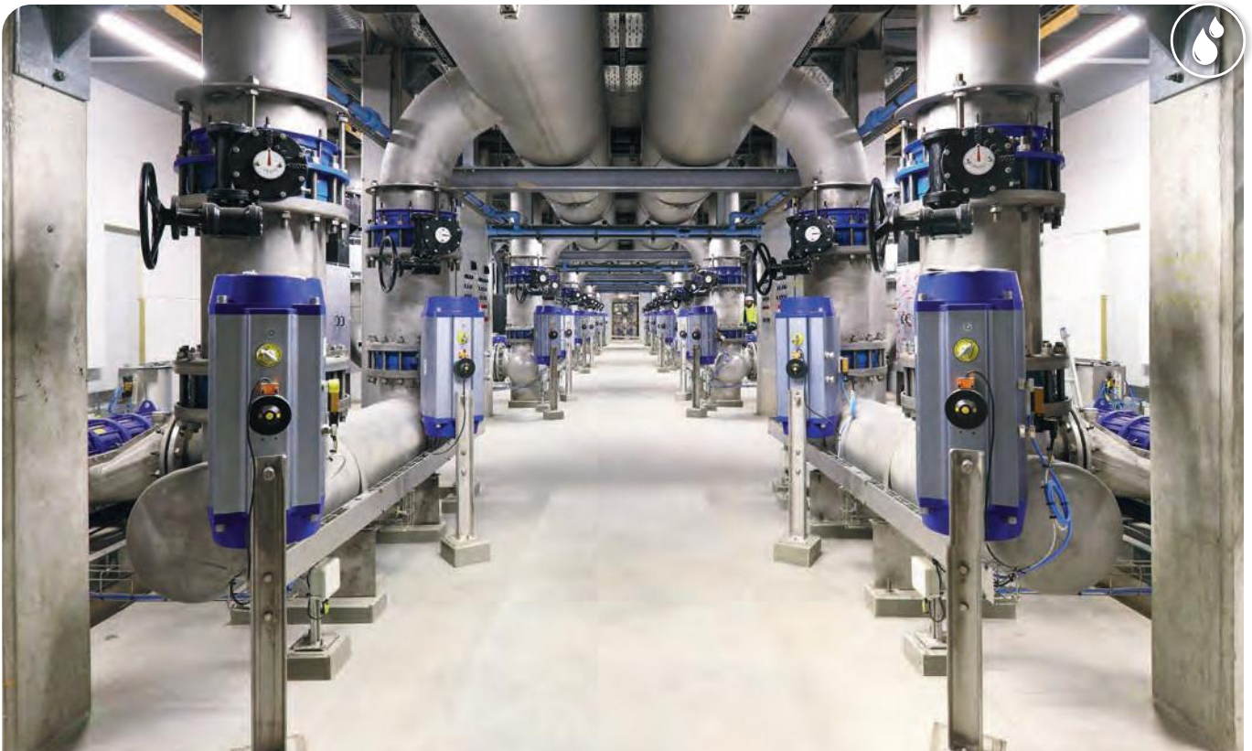
Station d'épuration | Eau | BELGIQUE Wastewater treatment plant - Water - BELGIUM
