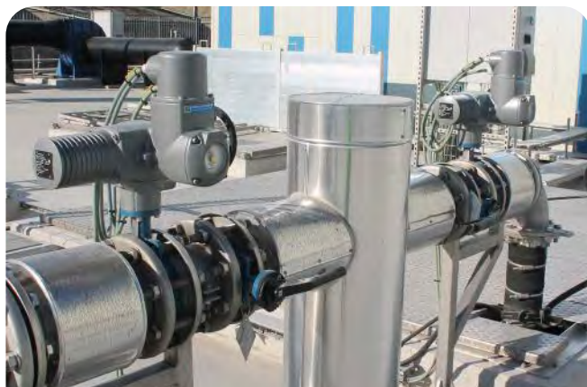
STEP | Eau | BELGIQUE WWTP | Water | BELGIUM
