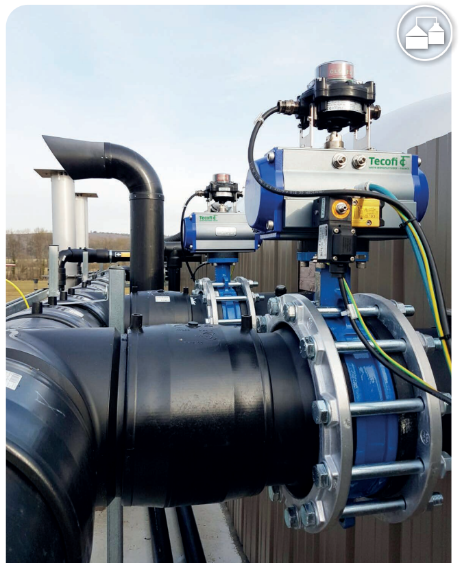
Biogaz | Industrie | FRANCE Biogas - FRANCE
