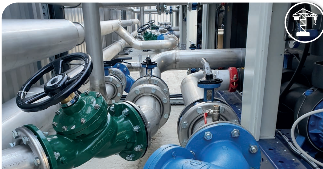
Chaufferie | HVAC | FRANCE Boiler Room - HVAC - FRANCE
